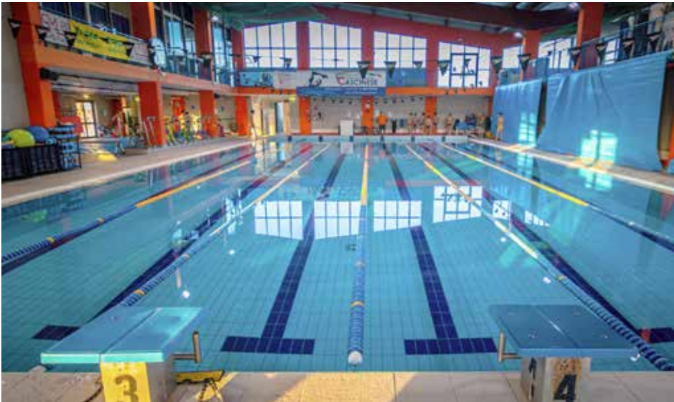
Cascina swimming pool (PI) Installation of energy recovery system
